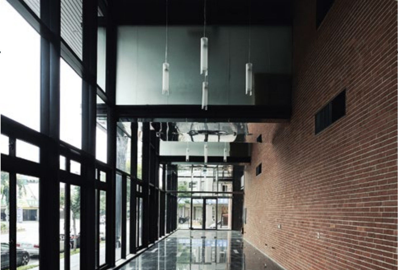
The glass wall on the lobby floor is a visual connection between the people inside and walkers on the pedestrian pathway.
