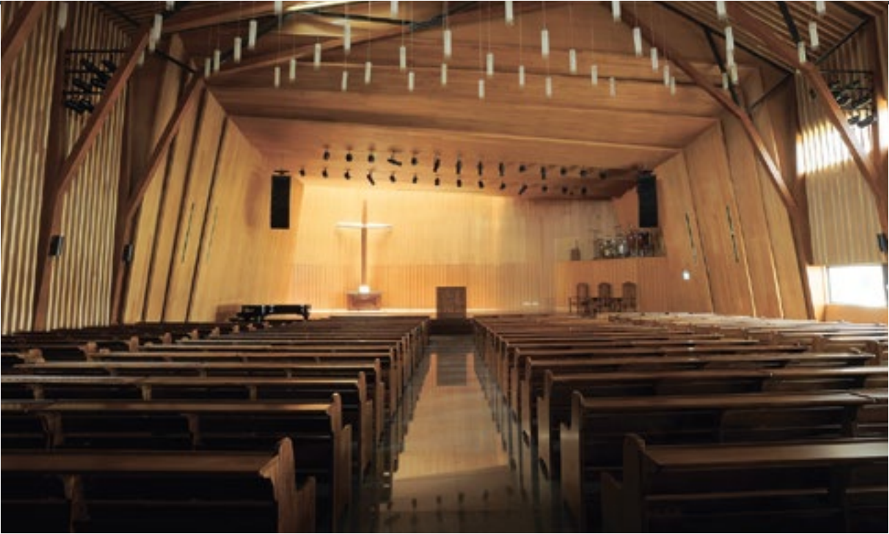
The worship hall is the most remarkable space in the church, with walls and ceilings featuring interrelated steel and wood in repeated hexagon shapes.
