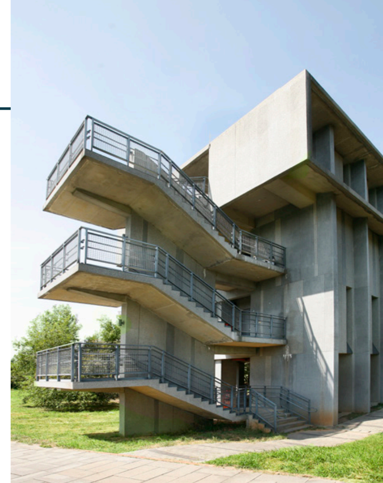
Structural elements such as pillars and poles are placed outside of the box-shaped exterior.
